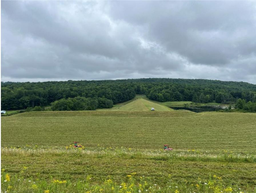
Chemung County Soil and Water performs Operation and Maintenance on five High Hazard Dams owned by Chemung County. The dams are mowed at least once a year and debris is removed from spillways on an ongoing basis. Inspections are coordinated with the Chemung County Buildings and Grounds, Chemung County Stormwater Coalition, The Department of Environmental Conservation Dam Safety and Natural Resource Conservation Service Watershed Operations.
