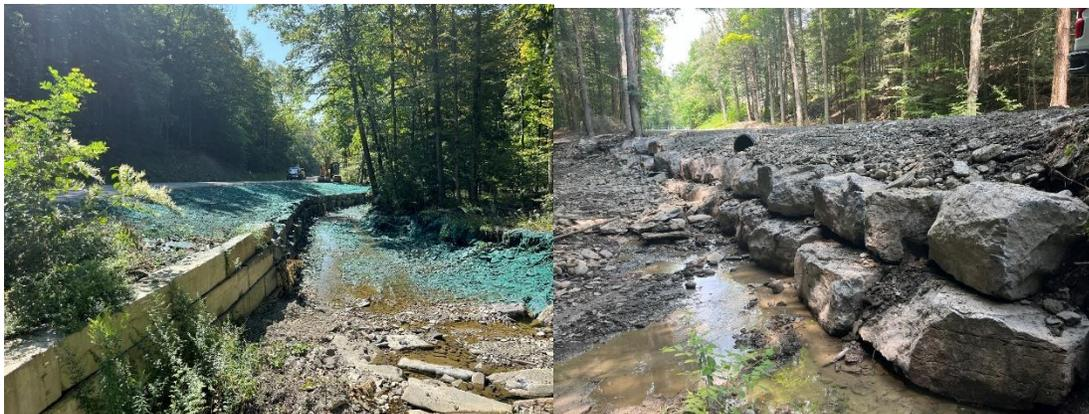
The Streambank team also worked alongside County DPW to replace a failing culvert along CR 60 with and upsized box culvert and install a DRY hydrant for use by the local Fire Dept.
