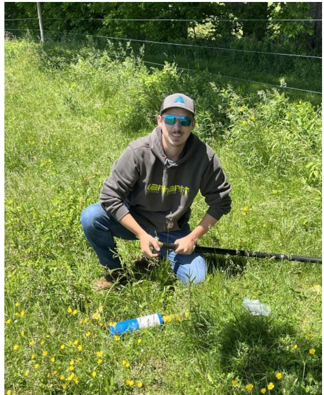
Tommy Conklin installing a pasture water system.
